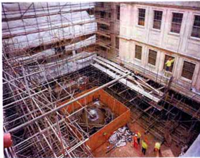
Left: major works in progress in the courtyard
