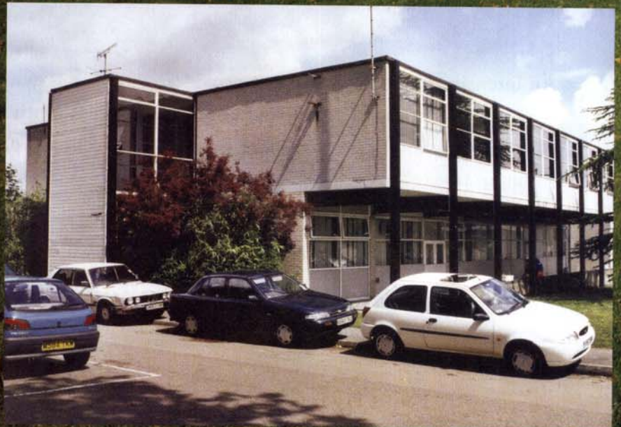
The college's front block has been extended to fill in the ground-floor set-back (see right). A new curtain wall has been added in keeping with the 1960s educational building
